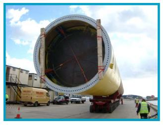
Plate 2.9 Pile, complete with tower flange, ready for loading
