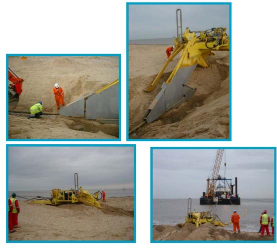
Plate 2.23 a-d Ploughed cable installation (across a beach with some pre-excavation in places)
